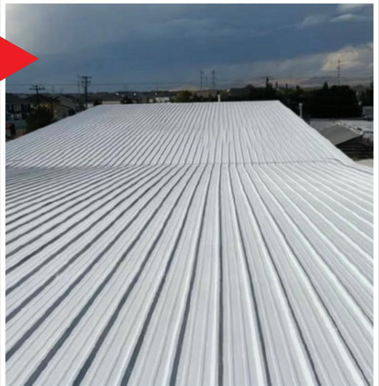
► The key difference is in the design and application – standing seam roofs take full advantage of having concealed fasteners. A standing seam system consists of wide, relatively flat metal panels that have vertical legs (or ribs) on each end.
